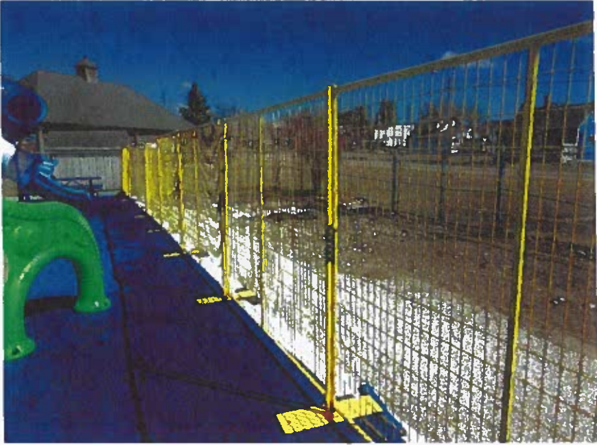
Temporary Construction Fencing
