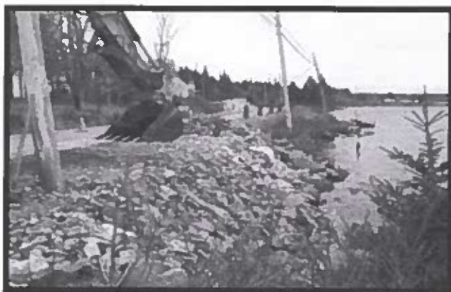
Brighton Road shouldering (2010)
