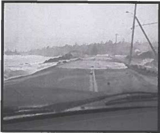
Locke Street West during storm surge Feb 2013
