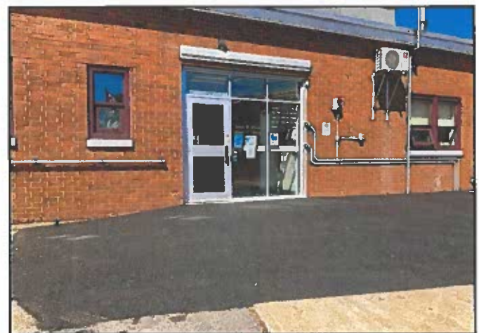
Digby library's new, accessible entrance is complete.
