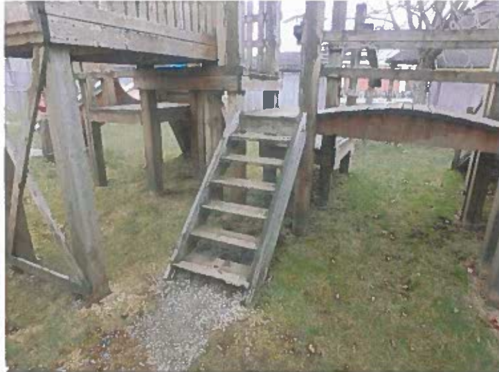
No Handrails on the Set of Stairs
