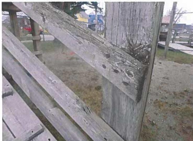
Nails Used to Fasten Wood Components
