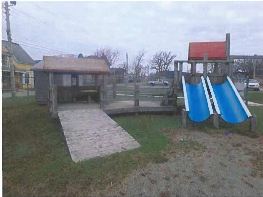
Structure View: Left Side
