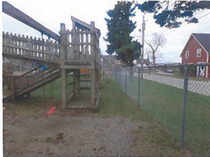
Non-Standard Protective Surfacing Zone
