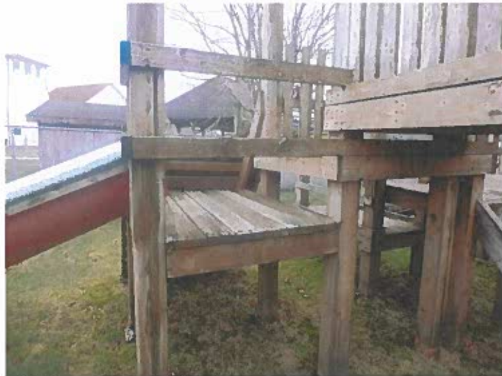
Non-Standard Platform for Half Tube Slide
