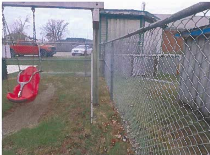
Non-Standard Clearance to the Side of Swing Set
