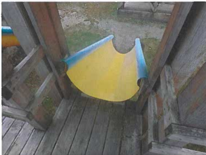
Non-Standard Platform for Half Tube Slide
