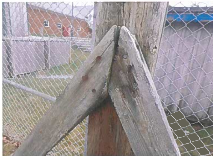
Nails Used to Connect Wood Components
