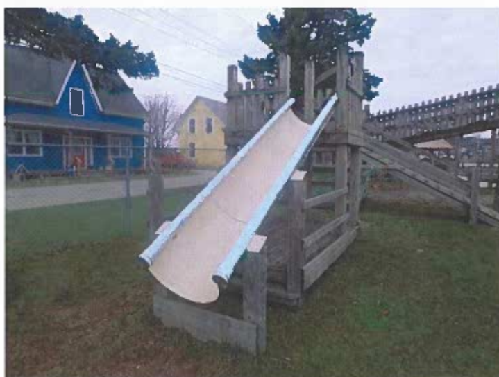
Non-standard Exit Area on Half Tube Slide
