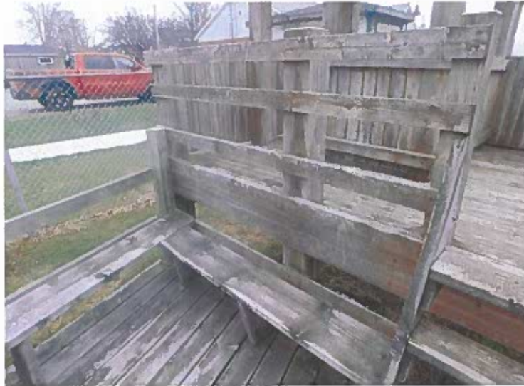
Head and Neck and Torso Entrapment Hazards
