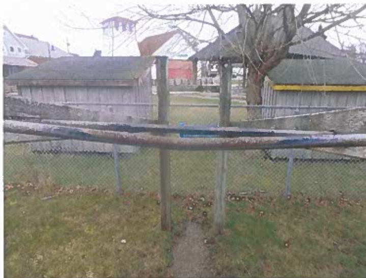
Bent Bar on Overhead Climber
