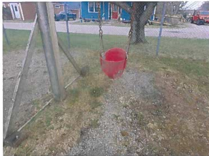
No Protective Surfacing Material
