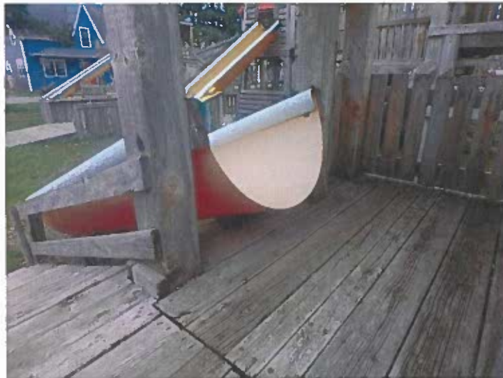
No Starting Platform for Half Tube Slide
