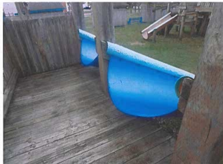
No Starting Platform for the Half Tube Slides
