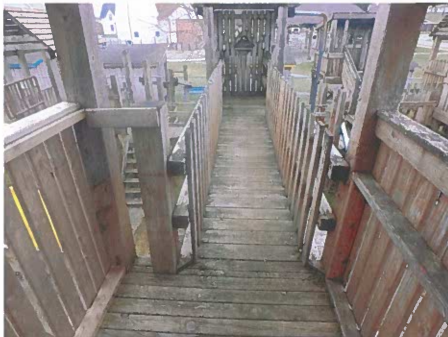
Elevated Platform Area
